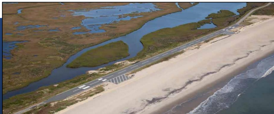
Wallops UAS runway located on Wallops Island: 1,500 feet long and 50-feet wide.
